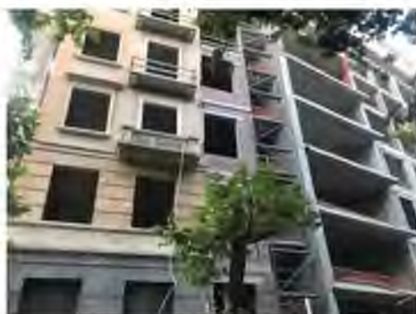
Photo 3. The process of combining the front and the new part
