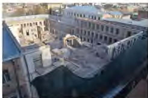
Photo 6. Reinforcing the facade walls and commencement of work
